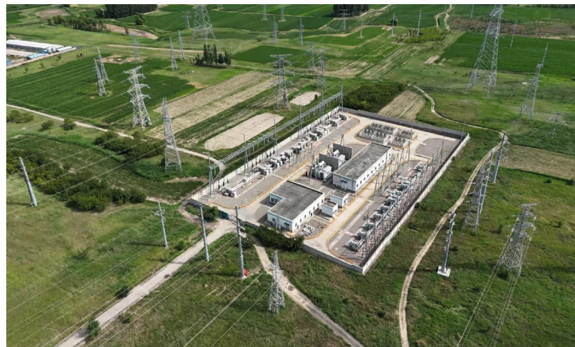
终点变电站现状
